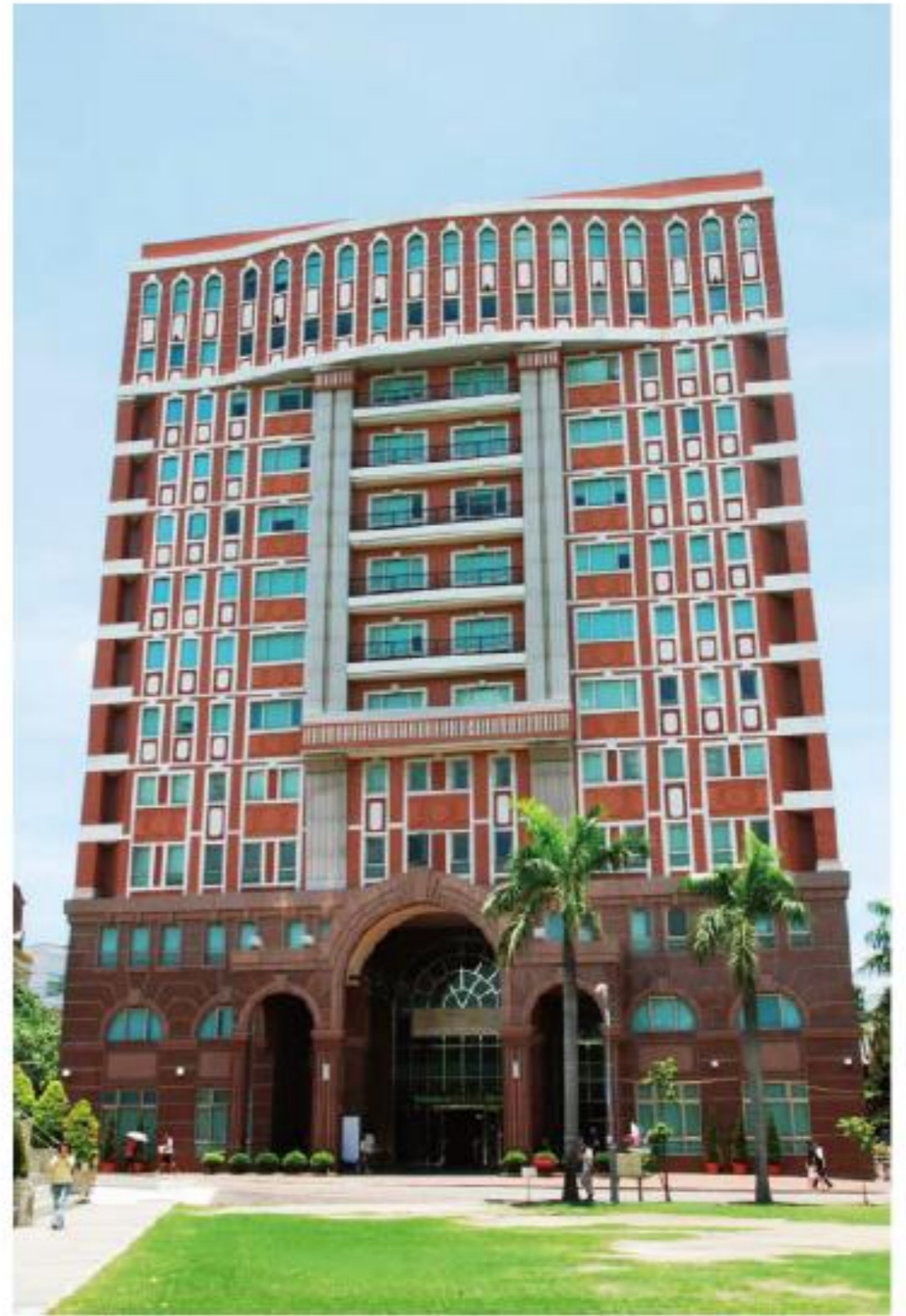
E Library and Information Building
